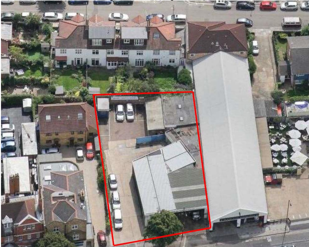
Fig 1- Aerial View looking south
